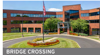
BRIDGE CROSSING US$43.3M Carrying Value (2) 100% Committed Occupancy
